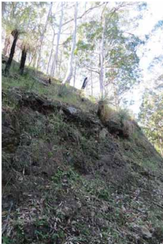
Figure 3.5 Soil creep occurring on several slopes along tracks in the general area of the Project
